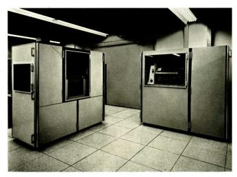
Unit Record Subsystem of large-scale L-3055 Data Processing System consists, in part, of a magnetic tape unit (below, left) used both as an input-output medium and as a repository for historical data. Some 256 such units can be accommodated.
