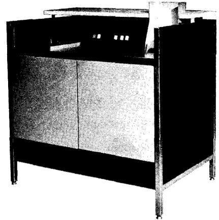
As shown in Figure 4-1, the basic components of the Type 214-1 Card Punch are an input hopper, a wait station, a punching station, and an output stacker. The input hopper has a capacity of 1,200 cards; the output stacker has a capacity of 1,300 cards. Cards may be loaded into the input hopper or removed from the output stacker during a punch operation. Selected cards or error cards may be offset-stacked in the output stacker.
