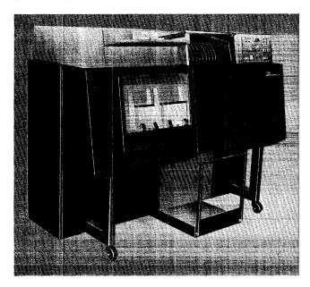
Figure H-12. IBM 1404 Printer, Model 2
