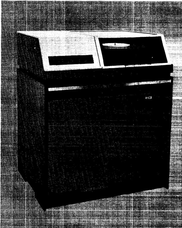
Figure G-15. IBM 1311 Disk Storage Drive
