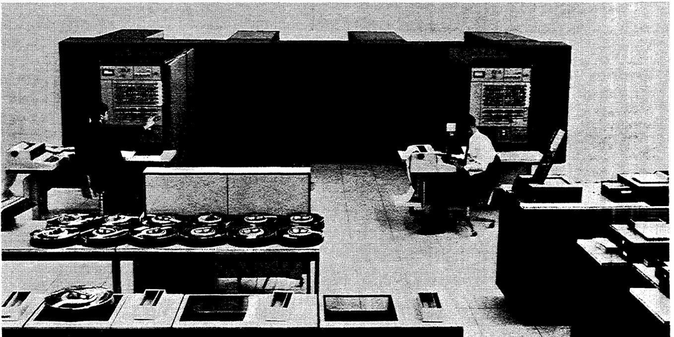
Figure 6-7. IBM System/360 Model 67-2 Duplex Configuration
