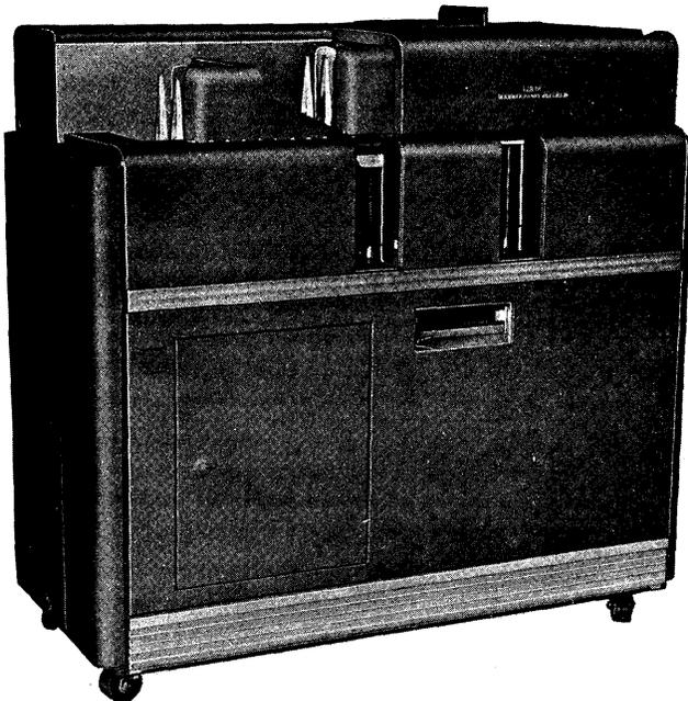
Figure 46. IBM 514 Reproducing Punch
