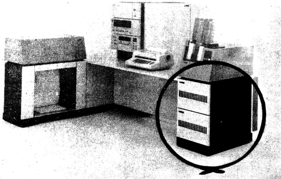
Figure 6-1. IBM 5444 Disk Storage Drive
