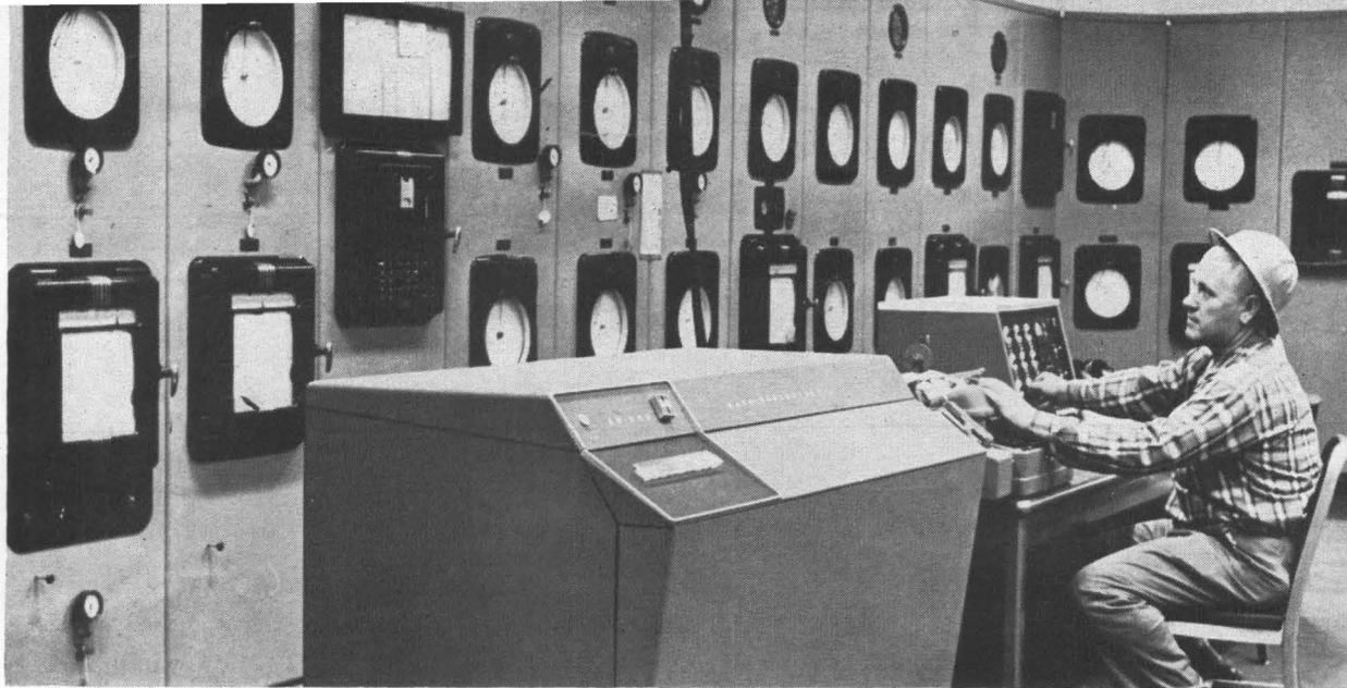
**Simulated** at Texas City were those instruments at the left next to the air gages. Tests using an RW-300 computer proved DDC'd loops responded at least as well as conventional loops but in most cases both smoother and faster
