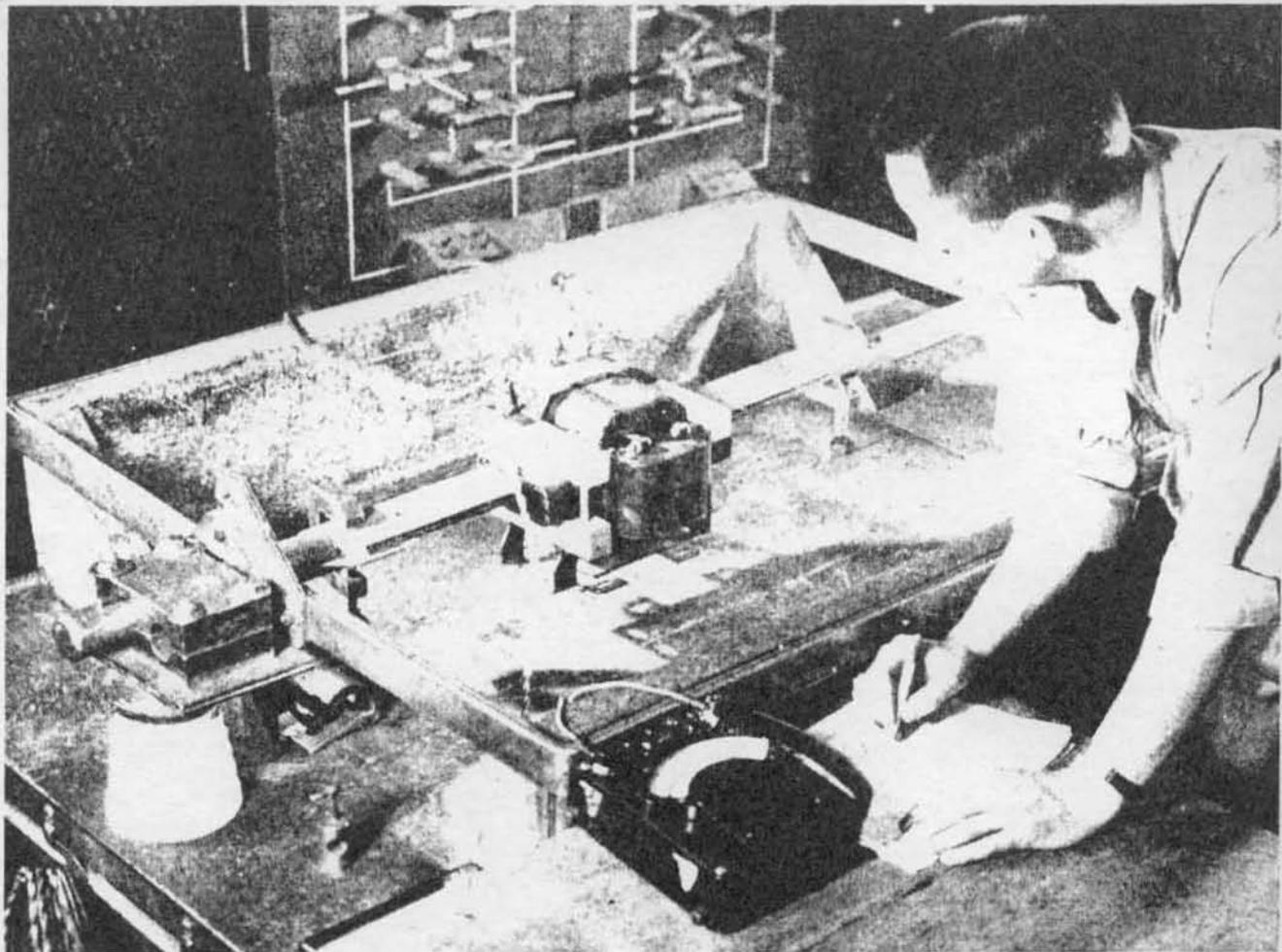
D-c current transductor under test. Device performs same function as a d-c shunt, however the metering circuit is electrically isolated, reducing hazard and amount of insulation required. Power dissipation is generally much less than in a comparable shunt.
