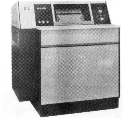
The UNIVAC 0768 Printer Subsystem is a freestanding, self-contained unit. The controlling and synchronizing circuitry, including the 132-character print buffer and the print mechanisms, are housed within the cabinet. This complete printer subsystem is connected to the UNIVAC 9480 System by means of the multiplexer channel. A separate multiplexer channel physical connection and shared subchannel address are required for each printer subsystem.
