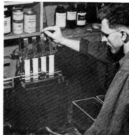
Figure 6 — A special developing tank with constant agitation assures correct development.
