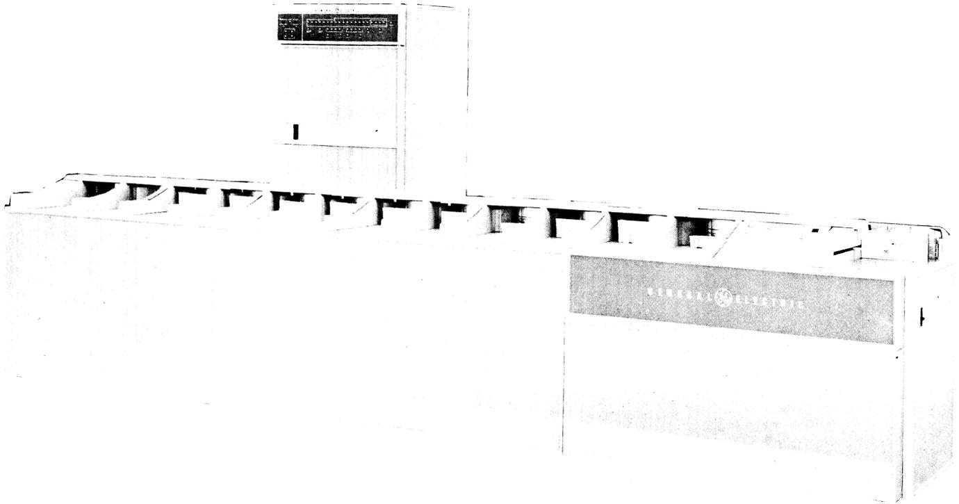
One or two DSU controllers can be connected to the controller selector; up to four DSU units can be connected to each controller. DSU reading and writing operations can proceed simultaneously with other peripheral and central processor operations.
