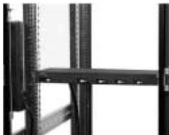
The modular PDUs have a unique modular architecture, and are designed specifically for the dense data center customers who want to maximize their power distribution and space efficiencies in the rack. Ranging from 16 to 40A models, the modular PDUs offer unprecedented flexibility, increased outlet receptacles (up to 32), easier accessibility, superior cable management and power distribution.
