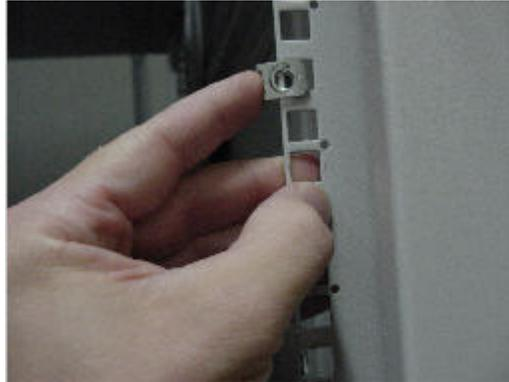
**Figure 7. Attaching Clipnuts to the Rack**
