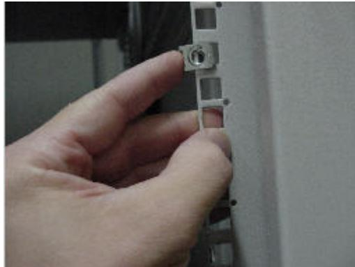
**Figure 17. Attaching Clipnuts to the Rack**
